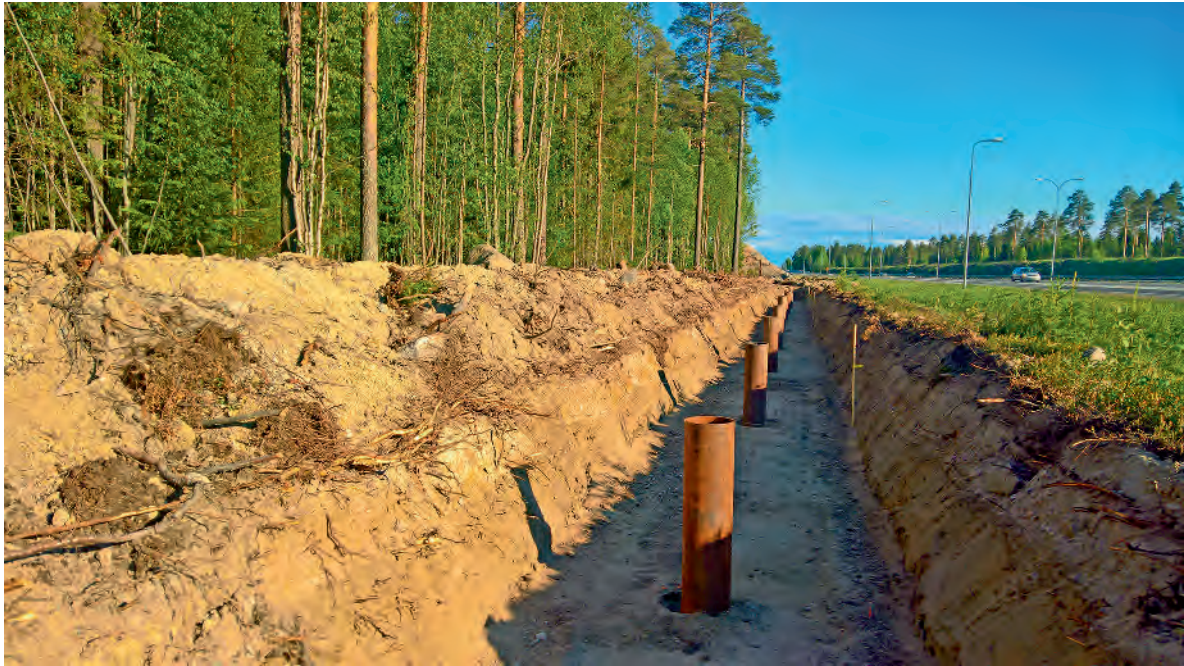
Figure 11.16. The foundation trench needed for the installation of a sound barrier caused a deep temporary scar on the western side of the Hiironen pet cemetery.
